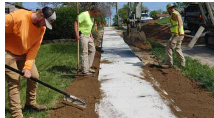
Construction of Rambling Hills Drive sidewalk this year
