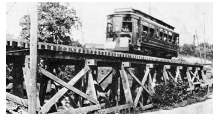
The IR&T trestle at Berkshire Road in Mt. Washington.
